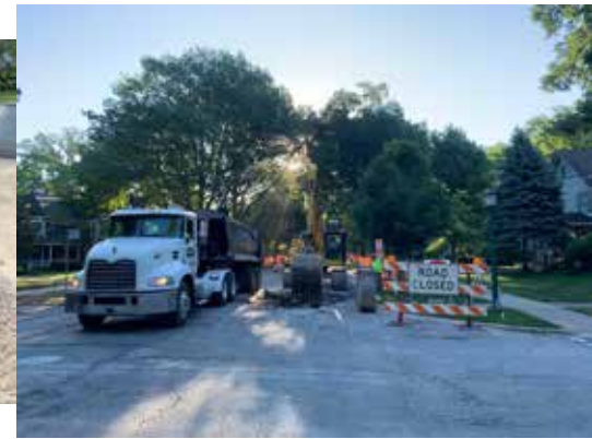
Watermain Work Along Central Avenue
