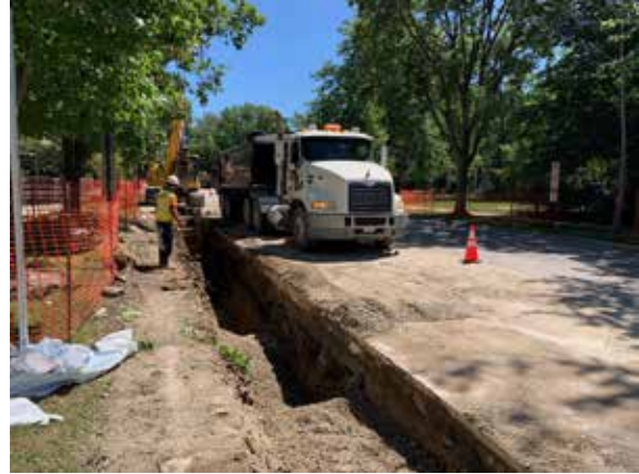
Watermain crew working near Central Elementary School.
